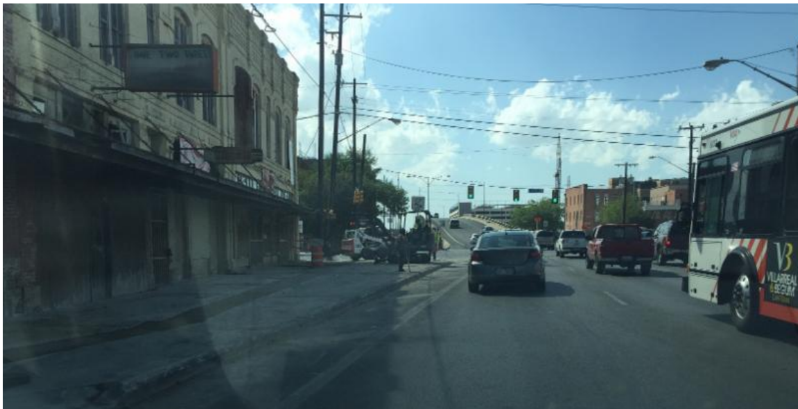
Gas work at Commerce
