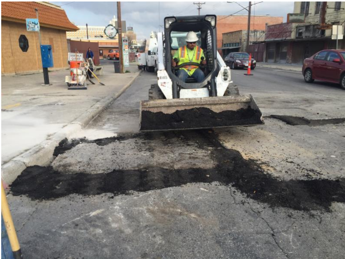
Gas work at Commerce
