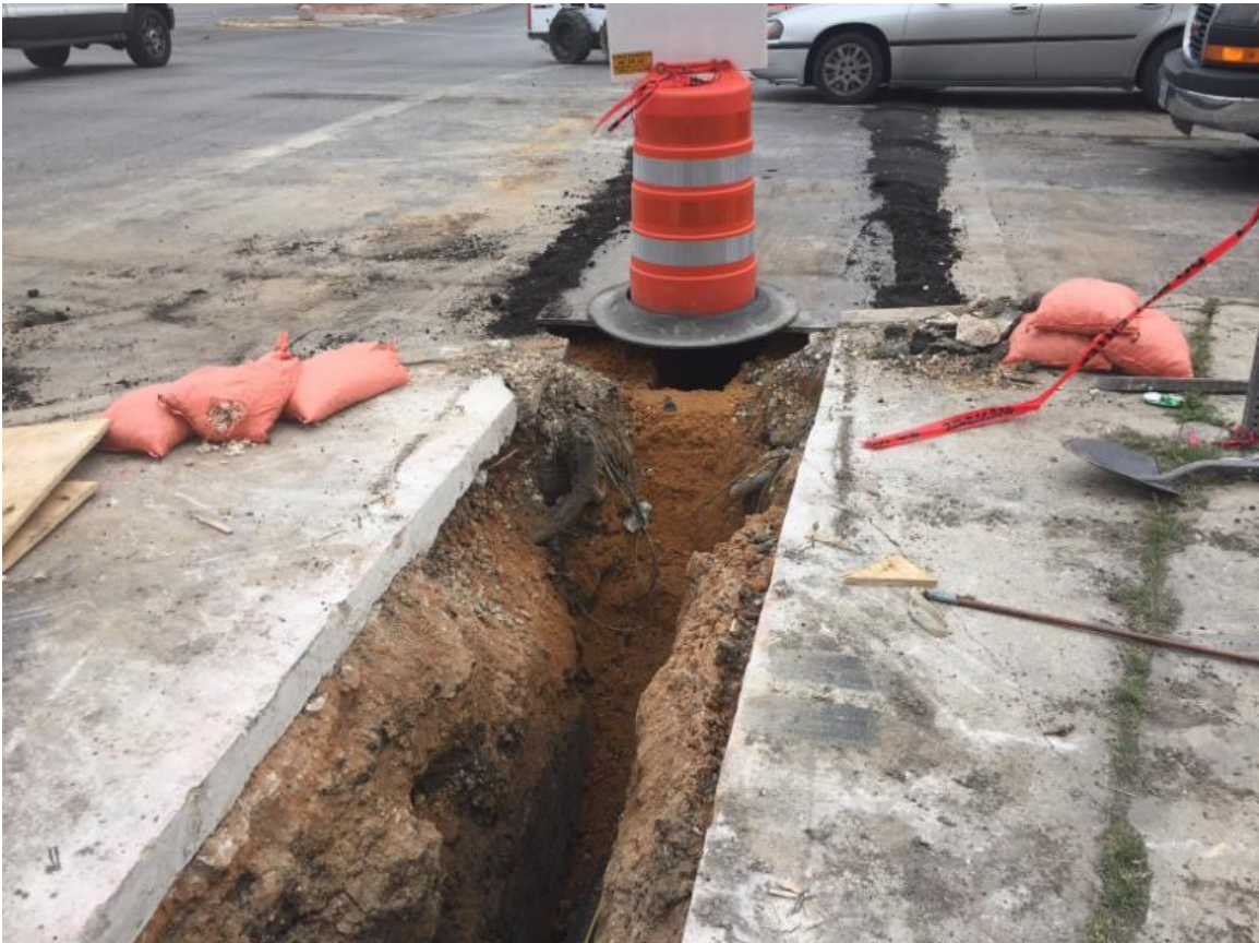
Trench for Gas installation
