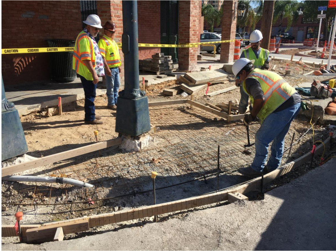
Sidewalk and wheel chair ramp forming at San Saba & Dolorosa
