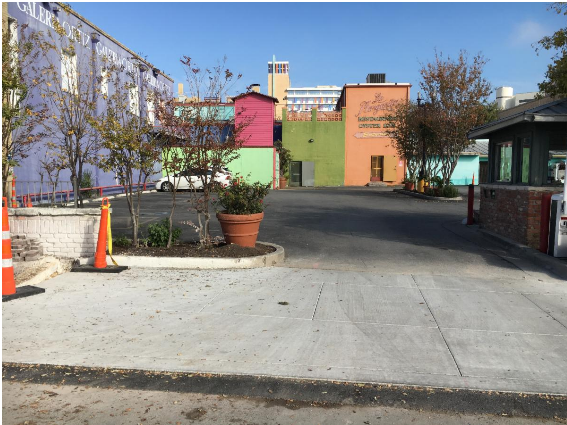
Completed driveway No. 4 at La Margarita
