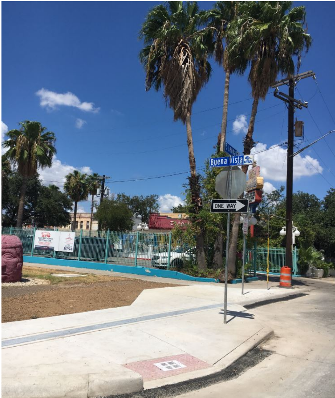
New curb, sidewalk and wheel chair ramps at Buena Vista & S. Leona northwest intersection
