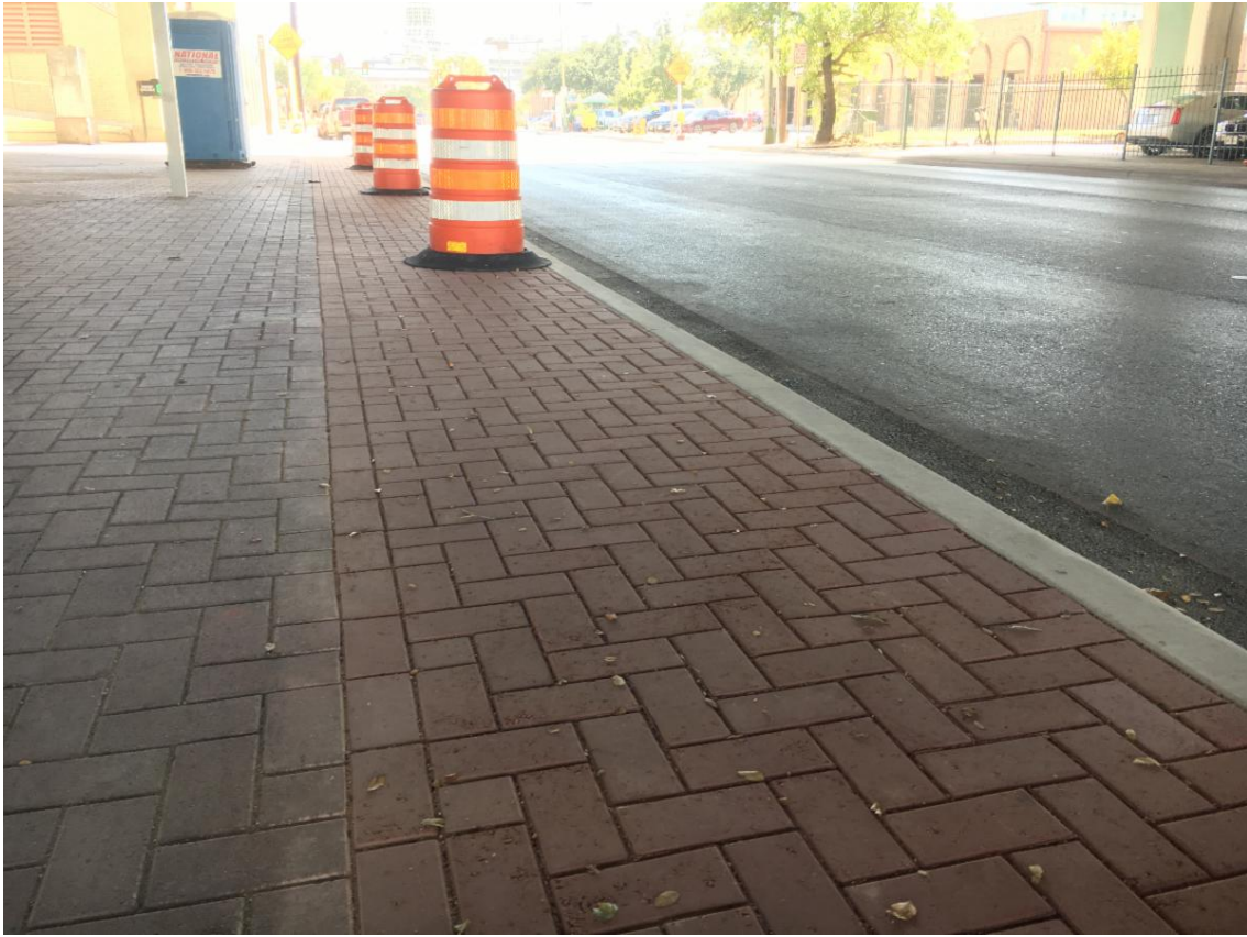
Brick pavers completed (Under IH-35)
