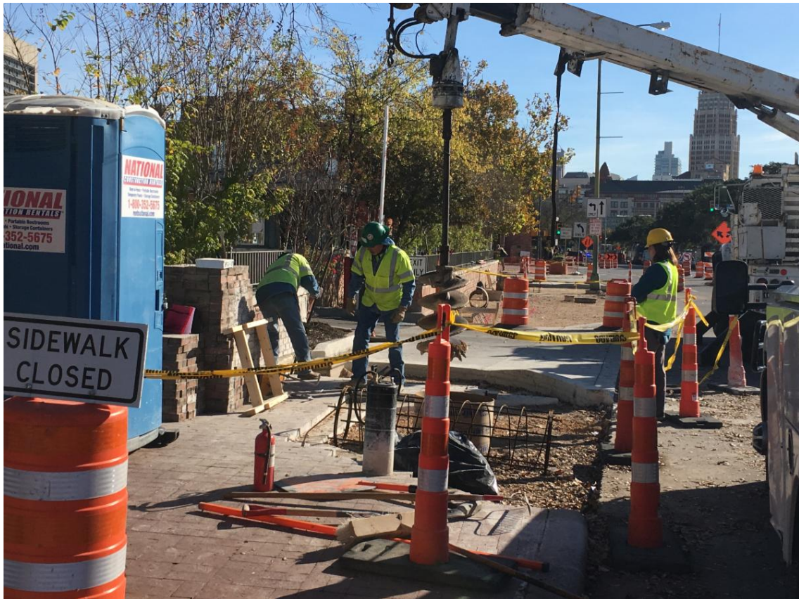
Drilling footings for pedestrian lights at La Margarita
