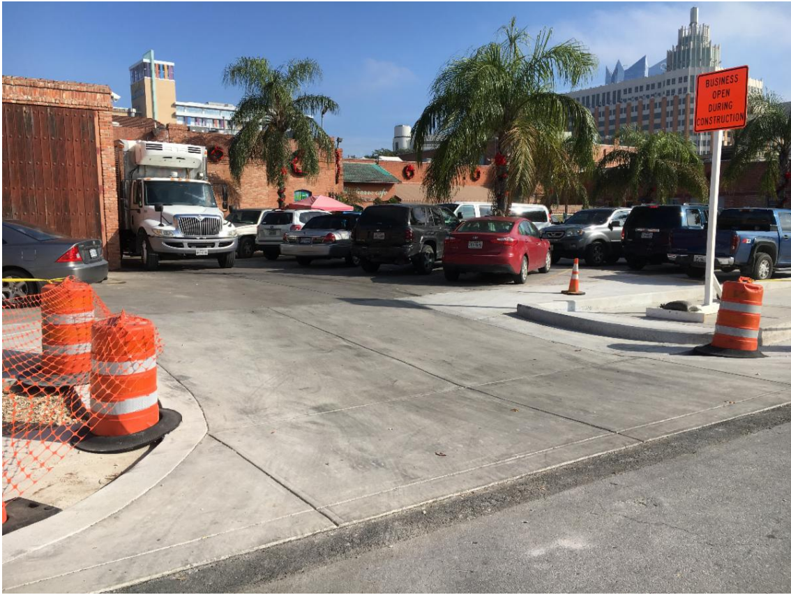
Completed driveway No. 1 at Mi Tierra
