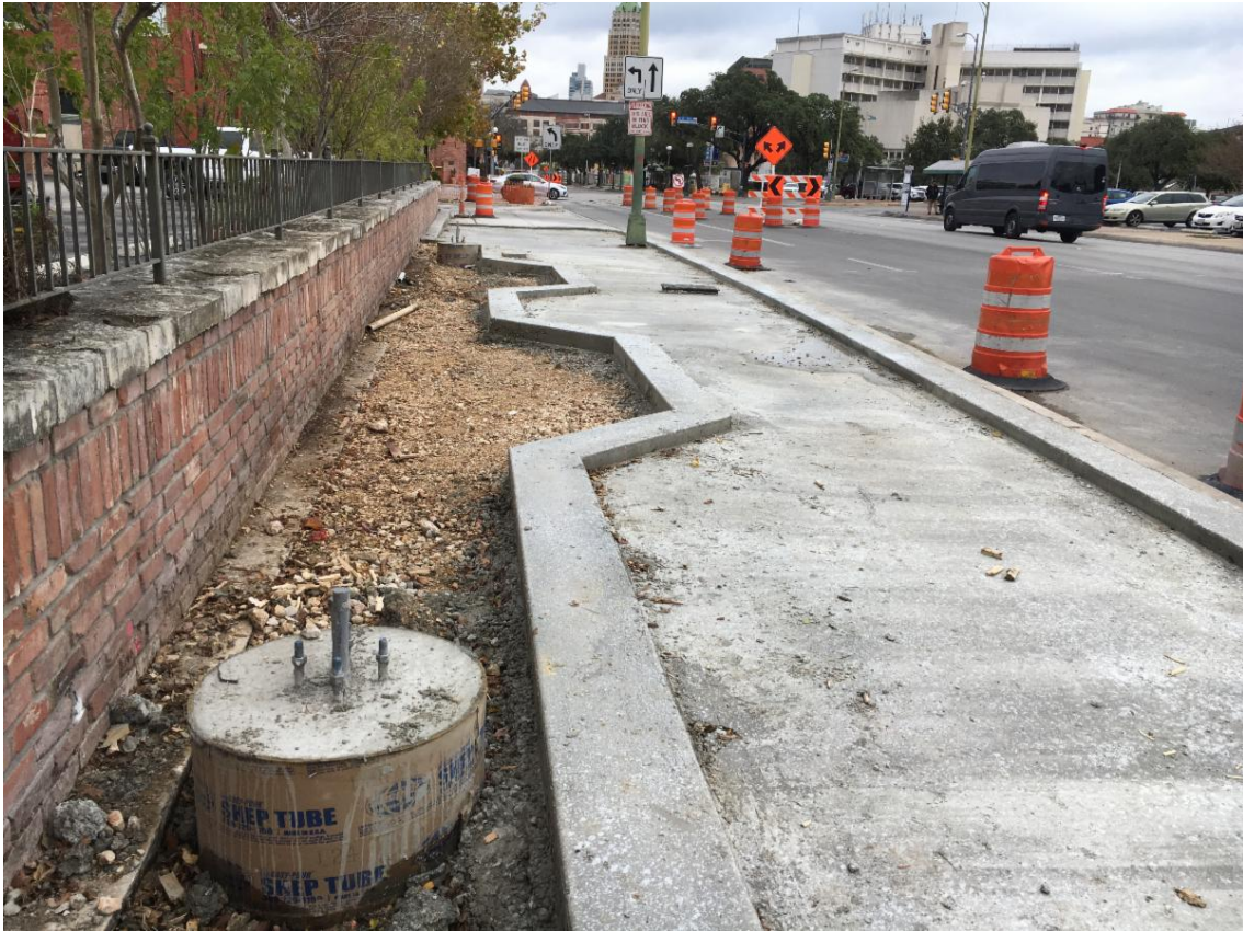
Preparing for brick pavers and pedestrian lights at La Margarita
